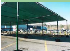
Garden Shade™ system at Walmart Garden Center
